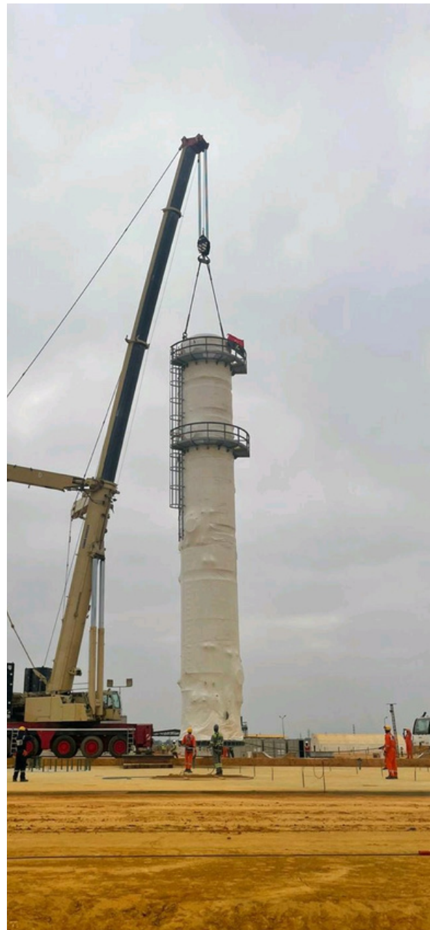
▲ VFuels' Crude Distillation Column D-100 was successfully installed at the site of the future 30,000 bpd Cabinda Refinery in Angola in June 2022.
